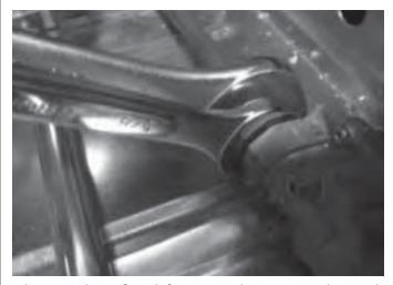
Always tighten flared fittings with two wrenches with opposing torque and do not over tighten. Using only one wrench or over tightening can cause leaks. Have someone stand by to close the main propane tank valve(s) while you are tightening fittings in case a leak occurs. After tightening, check again with the leak detection solution to be sure the leak is stopped. If bubbles still appear, your dealer or a gas service center may need to fix the problem.
