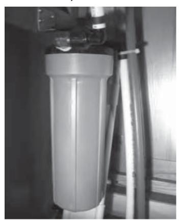
Many water filters are designed to remove sediment and particles from the water. Removing sediment and
