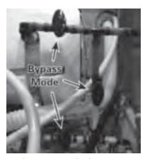
If the bypass valve is set to the bypass position, the water heater will not fill with water. If you don't get hot water after a reasonable time, check this valve and be sure it is set to the normal position.
