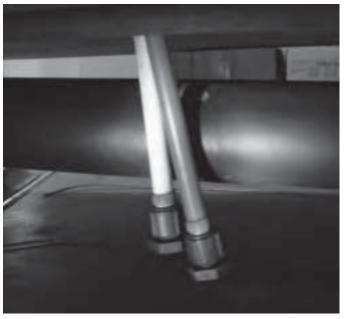
Open the system low point drain valves. These are the lowest points in the water system. The low point drains are located under the trailer. Drain out all water. Close the low point valves when ALL water is drained.
