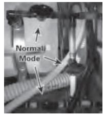
For normal water heater operation, be sure the bypass valve handle is set as shown above. To bypass the water heater for winterization, turn the valve handle one-quarter turn clockwise as shown below. The valve is a quarter-turn valve, and only has two positions — open and closed.
