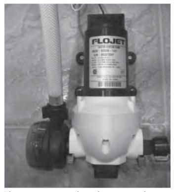
The water pump is a demand type pump that runs when a pressure drop in the water lines is detected, such as when a faucet is opened. The pump will continue to run until the faucet is closed and the pressure
