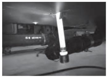
2. Turn the water heater OFF. Allow the heater to cool. Drain the water heater by removing the drain plug.
